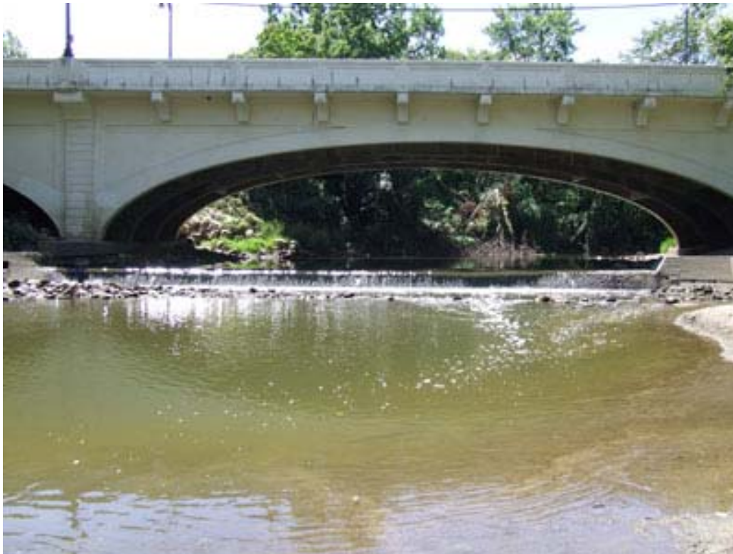
Photo 1: Highland Park dam and South Ave. bridge.
