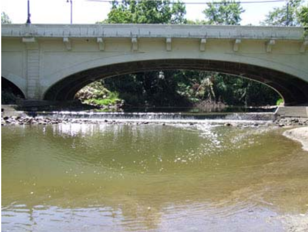
Photo 1: Highland Park dam and South Ave. bridge.
