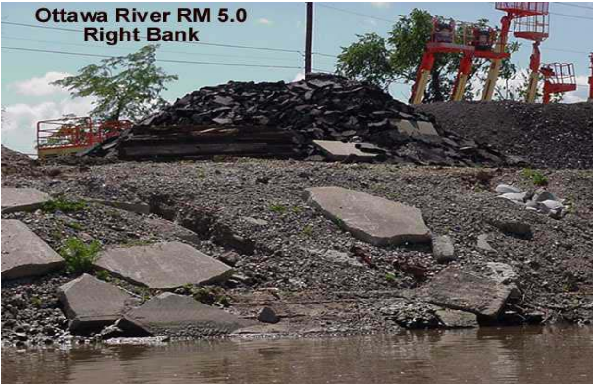
Figure 2-1 Right Bank of Ottawa River at River Mile 5.0
