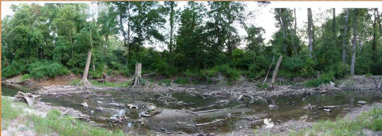
Address severe stream bank erosion
